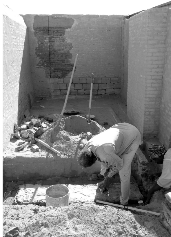
Fig. 19: Construction of the new outlet channel for the drainage of the site museum; note the re-modeled, though still unplastered area of the crack in the enclosure wall in the rear (photo: Claudia Näser)
