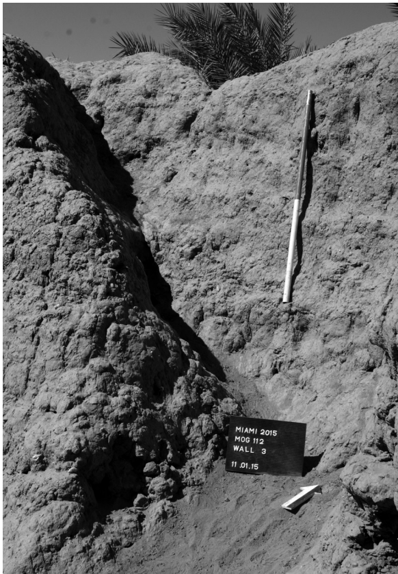
Fig. 29: Remains of staircase at northeastern end of the northwest wall of al-Hilla fortress, facing north (photo: Lisa Seelau)
