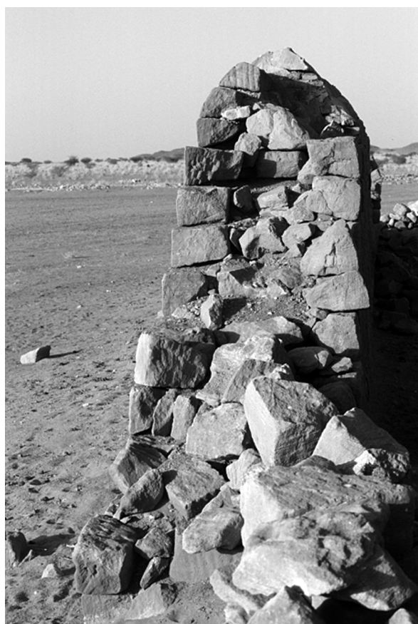
Fig. 5a: Section through wall 601/512, Building Period 6 (Hintze). Blocks of local sandstone in the shape of a truncated pyramid form the outer shell of walls. The core of the wall consists of sandstone rubble and earth mortar. No coat of plaster.
