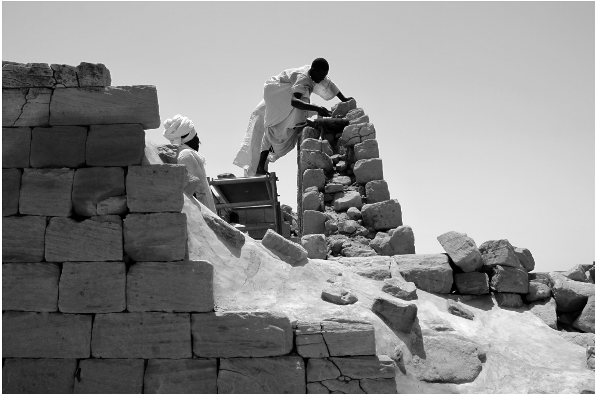
Fig. 14: Applying a lime mortar covering to an open wall top in Complex 200; in the foreground a wall top after treatment (photograph: Juliette Brauer and Franziska Lehmann)
