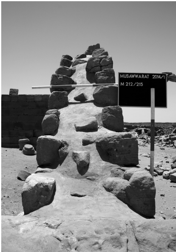
Fig. 15: Wall 212/215 with the protective cover of lime mortar in place (photograph: Juliette Brauer and Franziska Lehmann)
