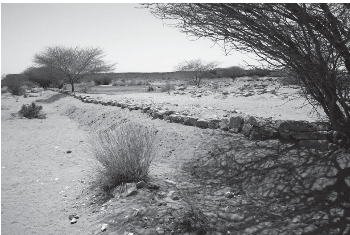
Fig. 10: The area east of the Great Enclosure with the rubble and earth platform and the newly constructed wall, covered by sand and equipped with a bank of sand on the wadi side (photograph: Cornelia Kleinitz)
