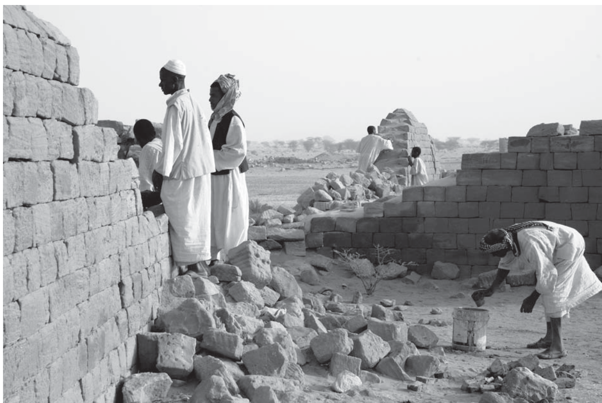
Fig. 22: Covering open wall tops with a lime mortar capping in Complex 500; in the centre and the background walls after treatment (photo: Claudia Näser)
