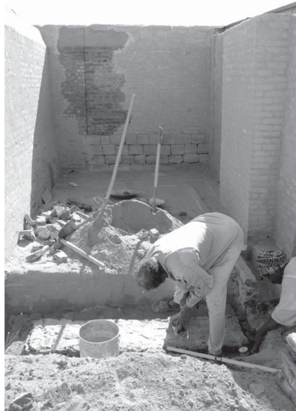
Fig. 19: Construction of the new outlet channel for the drainage of the site museum; note the re-modeled, though still unplastered area of the crack in the enclosure wall in the rear (photo: Claudia Näser)
