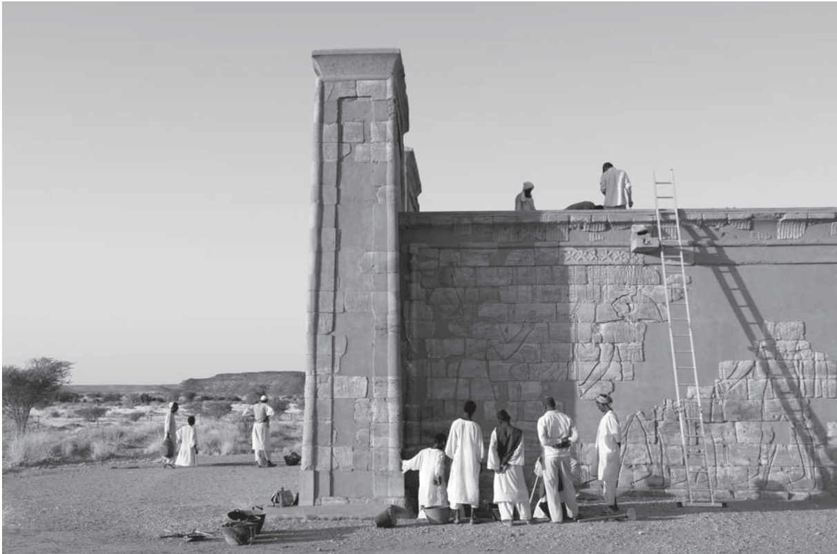
Fig. 4: Excavations at the southern and northern pylon towers of the Lion Temple, October 2014 (photo: Claudia Näser)
