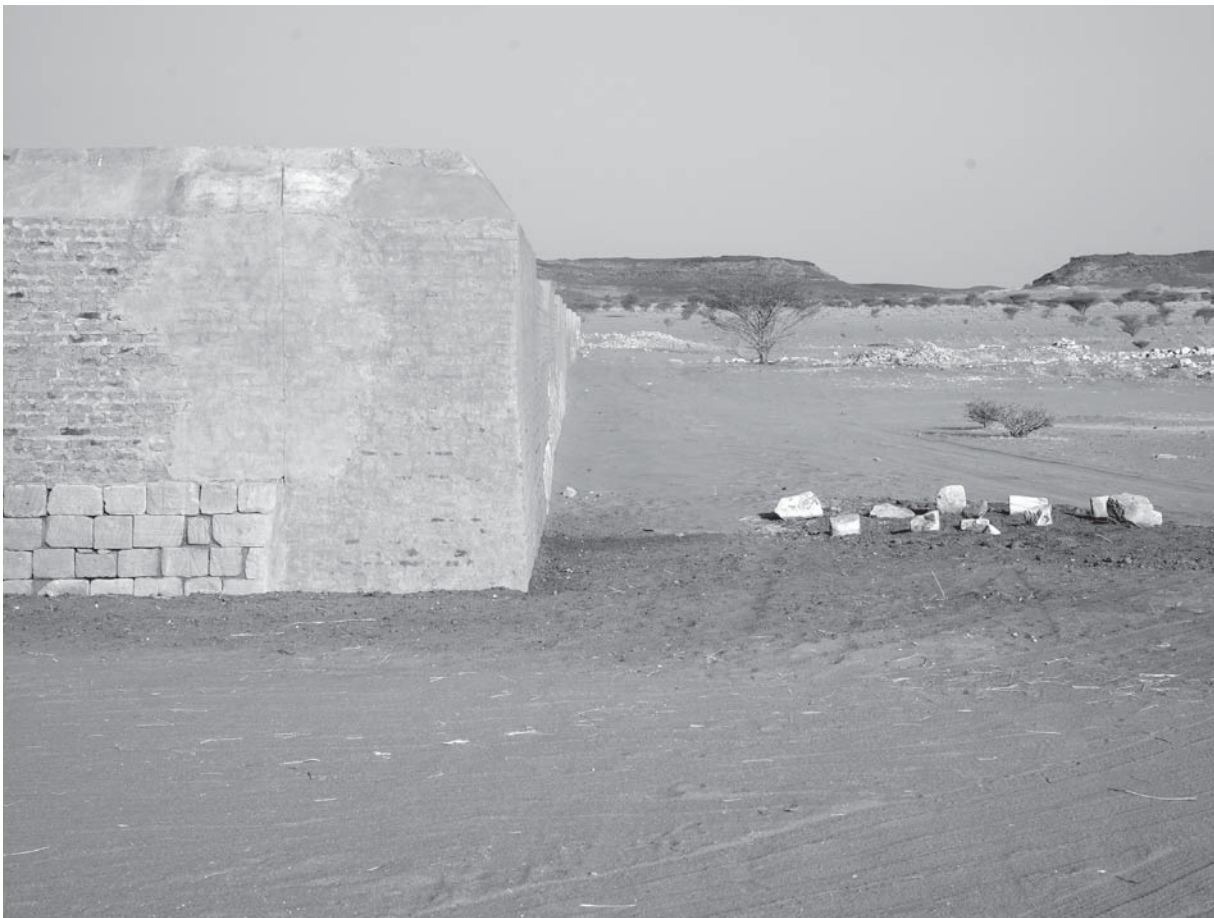
Fig. 21: The northeastern corner of the Great Enclosure after the completion of the measure (photo: Claudia Näser)
