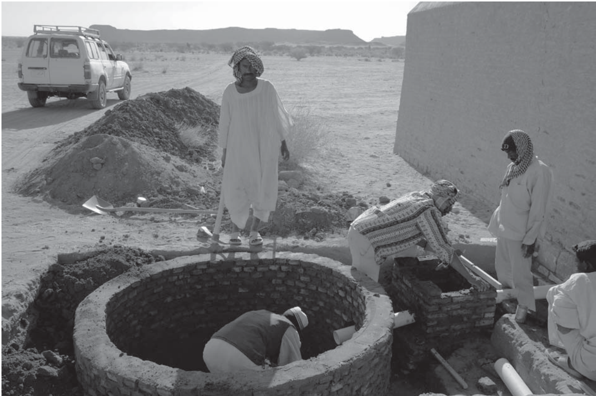
Fig. 20: Construction of the infiltration well outside the enclosure wall (photo: Claudia Näser)
