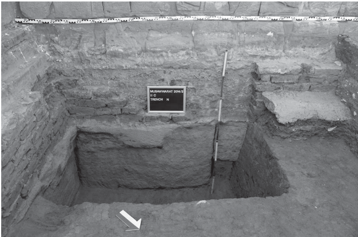
Fig. 5: The foundations of the reconstructed Lion Temple consisting of a mighty unreinforced concrete body underneath the actual reinforced concrete foundations, the brick-lining of which has been supported by a concrete 'shirt' (preserved on the right side), exposed in the trench in the rear of the northern pylon tower (photo: Claudia Näser)
