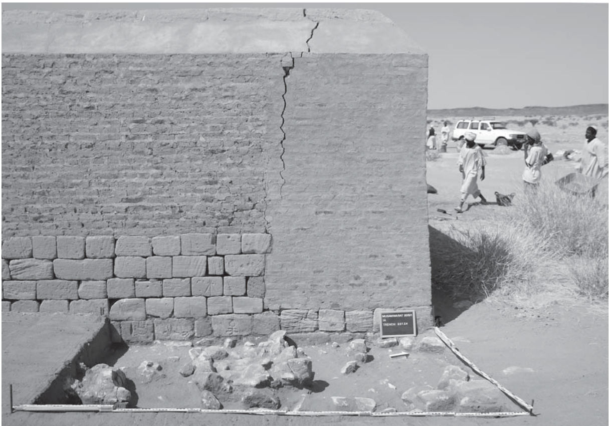
Fig. 18: Crack in the reconstructed enclosure wall at the northeastern corner of the Great Enclosure (photo: Claudia Näser)
