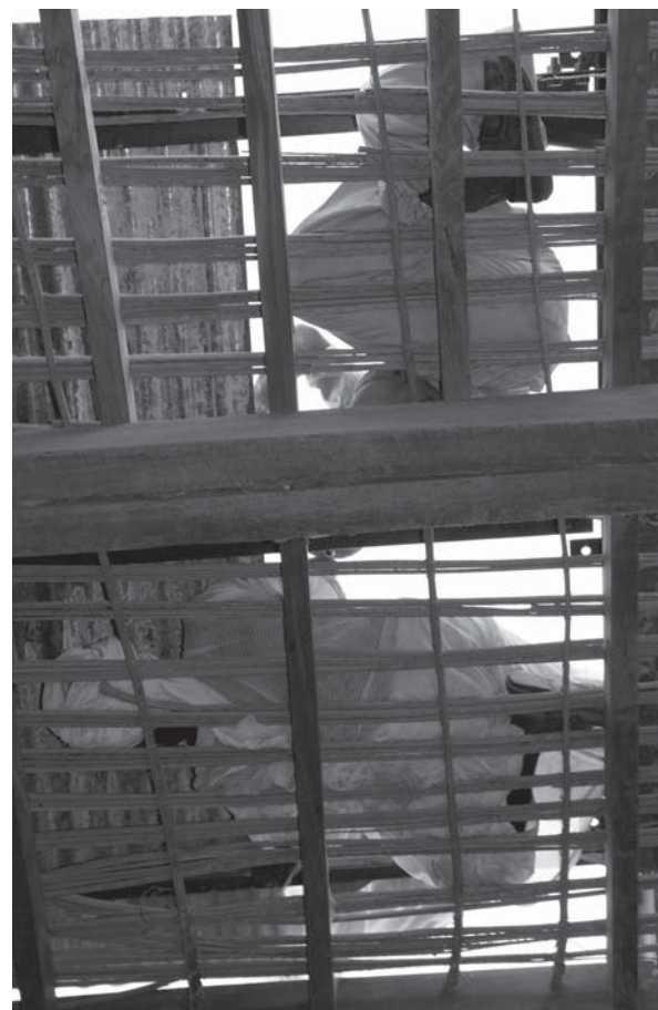
Fig. 3: Preparing the roof of the Lion Temple for investigation, October 2014 (photo: Claudia Näser)
