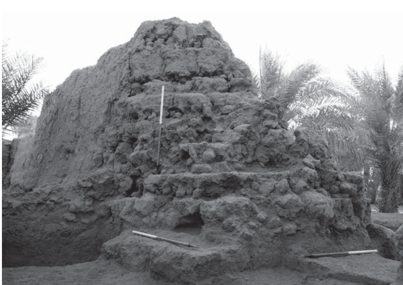
Fig. 32: Trench 2, showing construction method of the northwestern wall of al-Hilla fortress, facing east (photo: Garth Rees)
