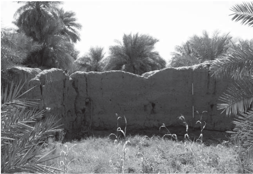
Fig. 28: The northwest wall of al-Hilla fortress during excavation of Trench 2, facing northwest (photo: Rizwan Ahmed)
